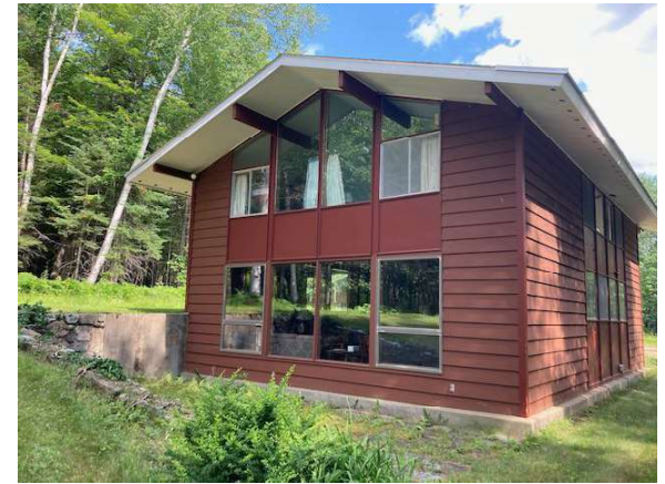
BEFORE | REAR VIEW
