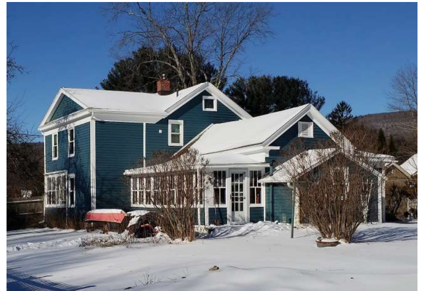
BEFORE | SOUTH EAST RENOVATION
