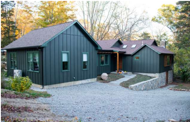
AFTER | FRONT VIEW
