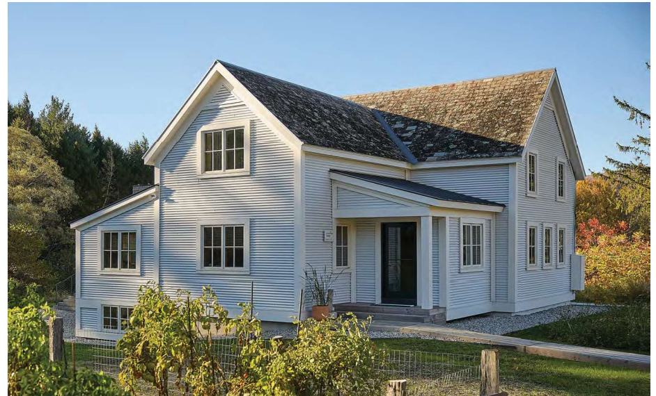
AFTER | FRONT VIEW PHOTO CREDITS: Will Russell
