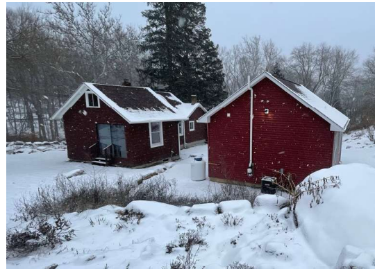
BEFORE | REAR VIEW
