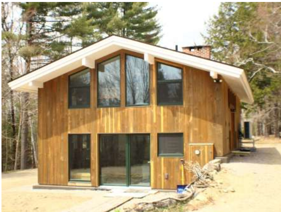
AFTER | FRONT VIEW
