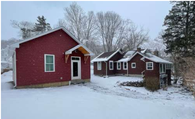
BEFORE | FRONT VIEW
