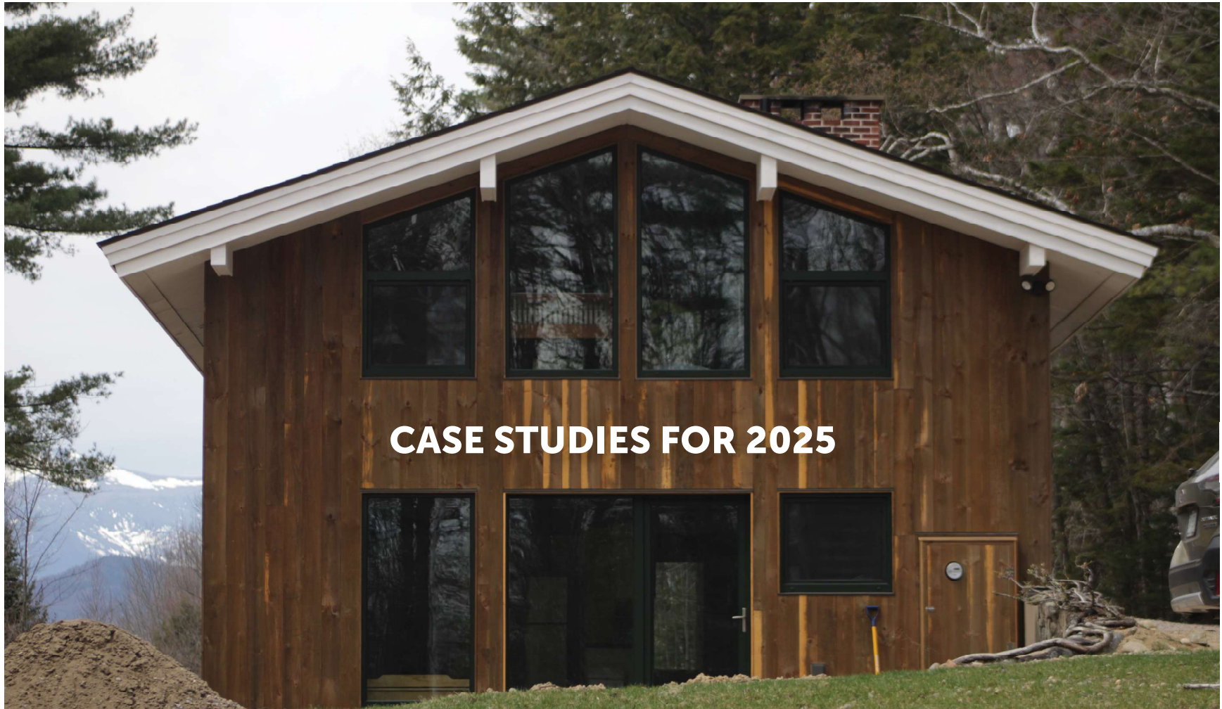
Abisalih Techbuilt Deep Energy Retrofit, Intervale, NH
