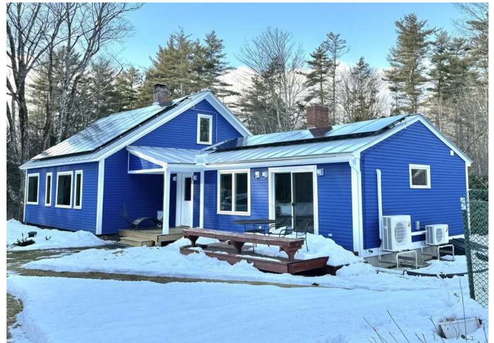
AFTER | EXTERIOR FRONT
