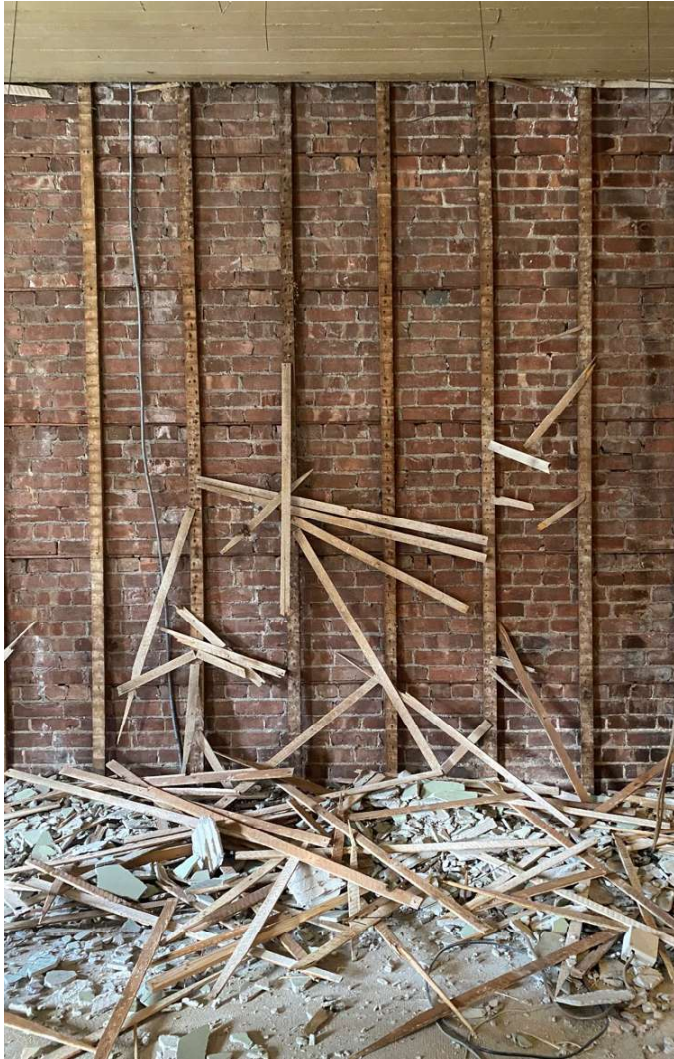
North River Electric House, Stone Ridge, NY
