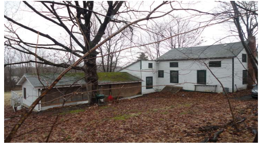
BEFORE | REAR VIEW
