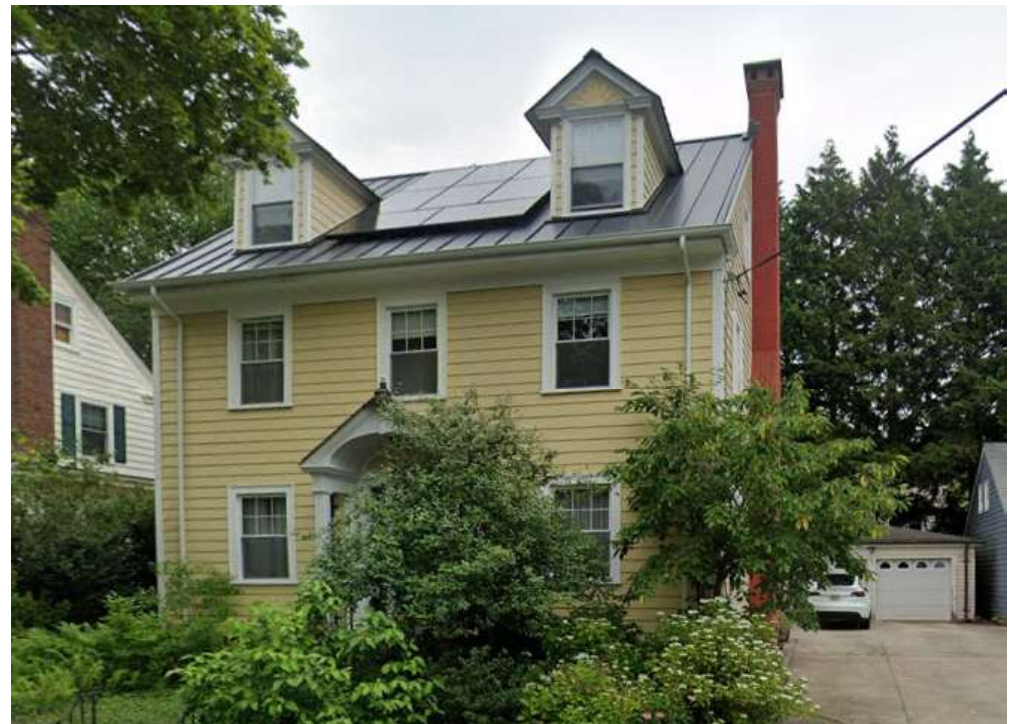
AFTER | FRONT VIEW
